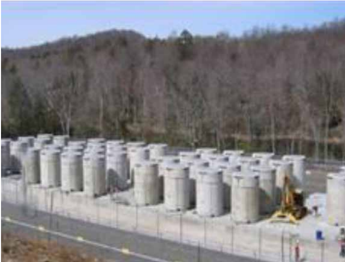
Dry cask storage for nuclear waste. Credit: U.S. NRC
