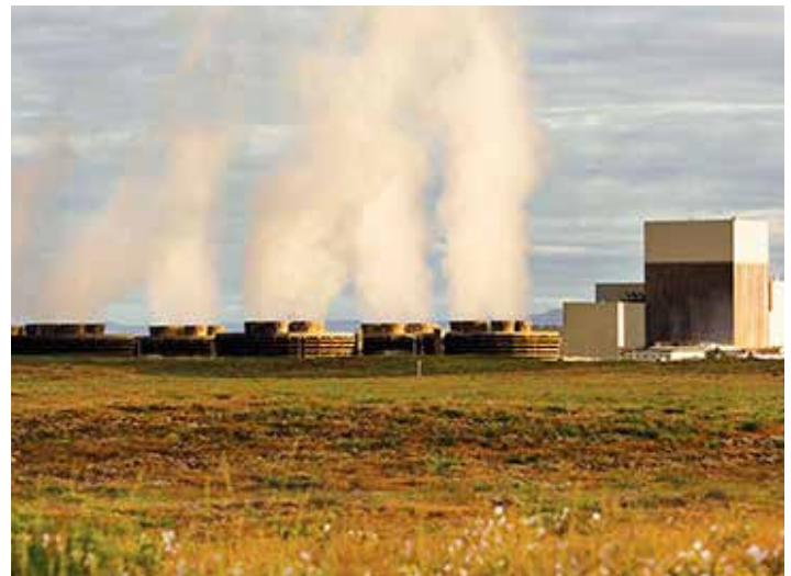
Columbia Generating Station. Credit: BPA
