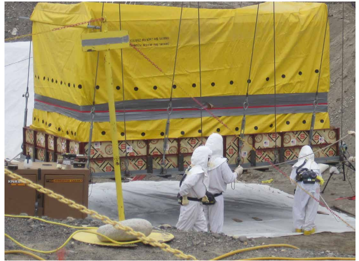
Workers remove a box of transuranic waste during current Hanford cleanup efforts. Credit: U.S. DOE
